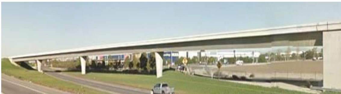
Figure 1. A view of the Fairview Road On-Ramp Overcrossing (FRO) Bridge
