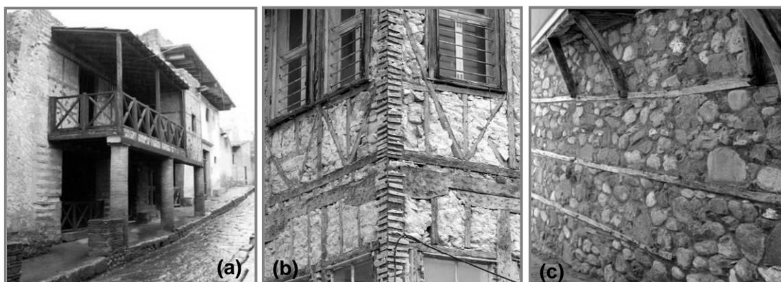
Figure 1: (a) Timber-Laced Masonry House from Herculaneum dating 78 A.D.), (b) Timber Laced Wall, (c) Stone masonry timber laced wall
