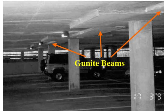
**Figure 7. Gunitite beams applied to the underside of the garage decks**
