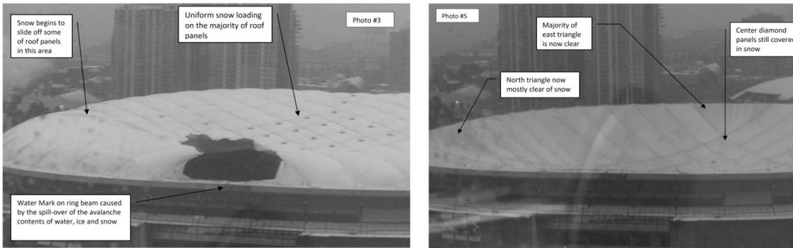
Figure 2: BC roof break (left) and deflation (right) [1]
