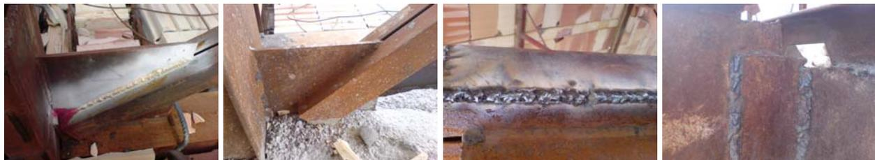
Figure 6. Some typical welding in the dormitory
