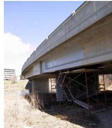
Figure 2. Shear strengthening of a concrete bridge girder
