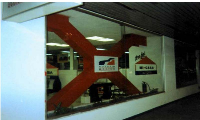
Figure 8. A reinforced concrete frame strengthened using a concentric steel brace.
