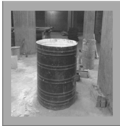
Fig 4 Container for Casting Concrete
