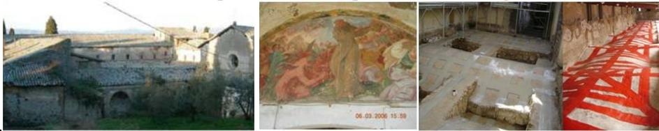
Figure 7. Retrofit of the masonry barrel and cross vaults with unidirectional GFRP sheets.
