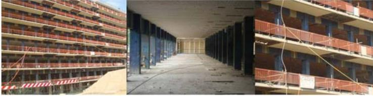
Figure 3. View of the concrete frame of the CTO Careggi hospital strengthened with CFRP sheets.
