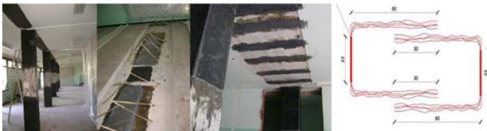
Figure 6. Overview of the additional stirrups made of UHTSS steel fiber sheet.
