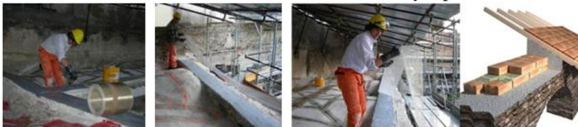
Figure 8. Strengthening of the ring corbel masonry beam with FID-Steel Hardwire®.
