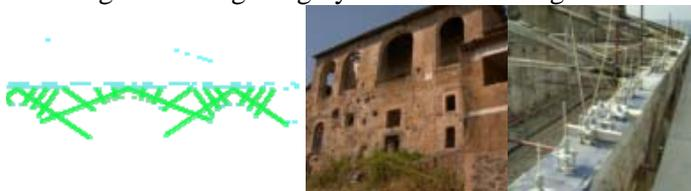
Figure 9. Strengthening of masonry arches using pretensioned FID-ASLAN 100 GFRP bars.
