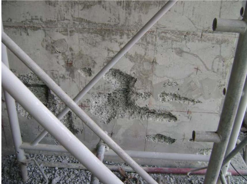
Figure 2. Surface damage at the bottom of the column.
