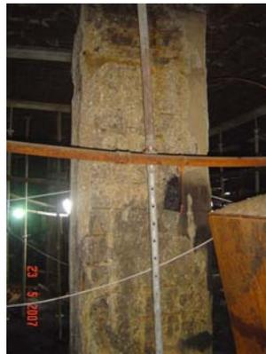
Figure 5. Buff colour observed on a concrete column.
