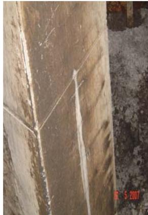
Figure 6. Extensive crazing on a column surface.
