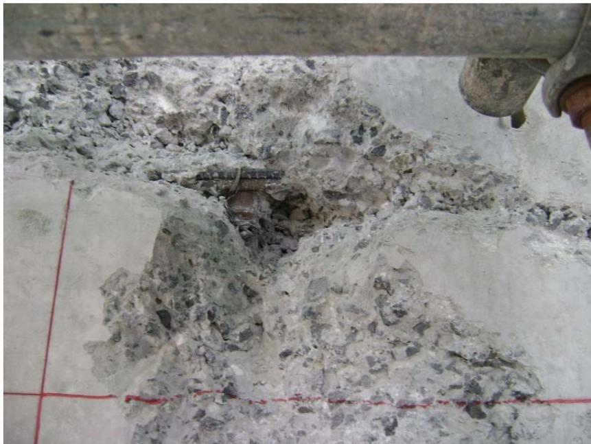
Figure 3. Exposed reinforcement due to poor consolidation of concrete.
