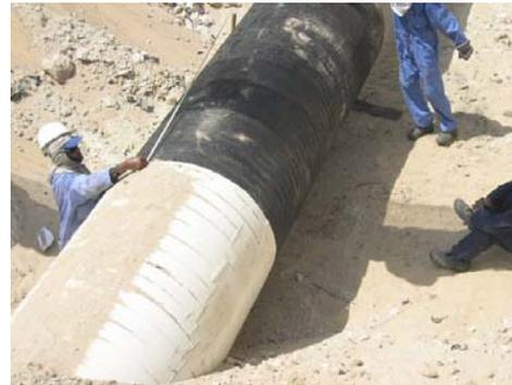
Figure 2. Instrumented 46" dia oil pipeline.
