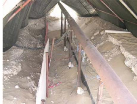
Figure 3. Buried pipeline exposed for fixing sensors.
