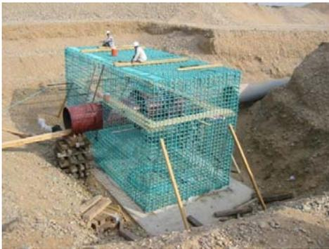
Figure 1. Concrete anchor block under construction.
