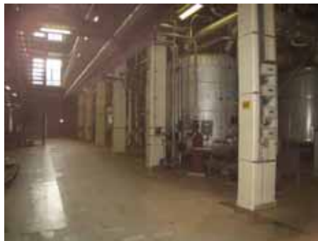
Fig. 2: Ground floor columns.
