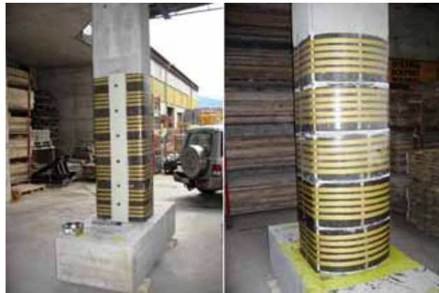
Fig. 4: Strengthening of columns P3 and P4.
