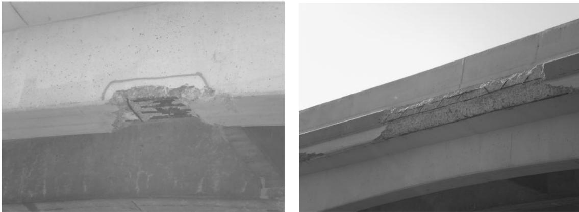
Figure 1. Damage caused by an overweight vehicle and spalling of concrete cover of a bridge girder.
