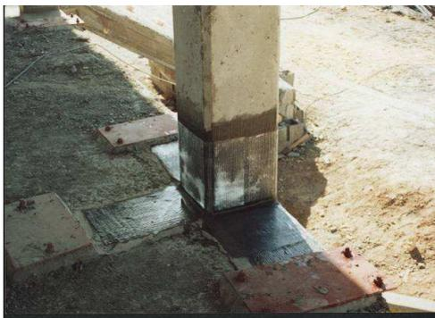
Column-beam connection by using FRP bands
