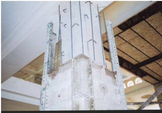
Installation of concrete jacket around column
