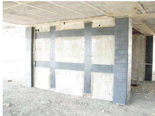
Adding shear wall and enforcing it with FRP bands
