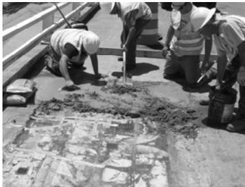
Figure 5. Concrete casting over area of bridge deck strengthened with FRP after installing strain gauges.
