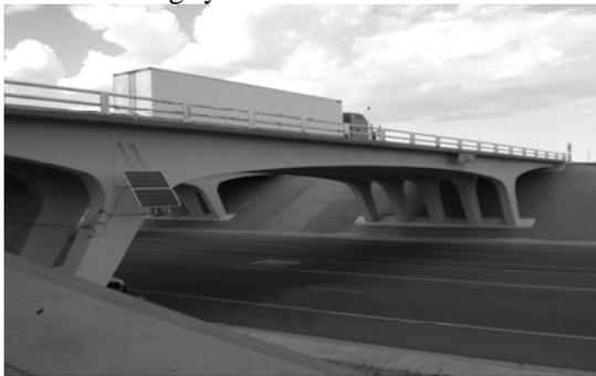
Figure 7. Solar power system installed on bridge 7937 provides clean renewable energy for SHM.
