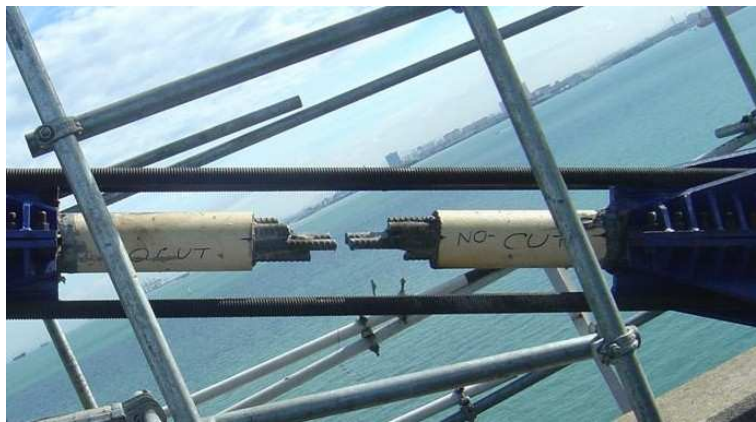
Fig 8 : controlled cable distressing in progress
