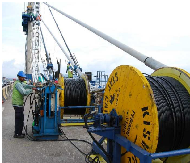
Fig 9 : Parallel strand stay cable installation on a bridge under traffic
