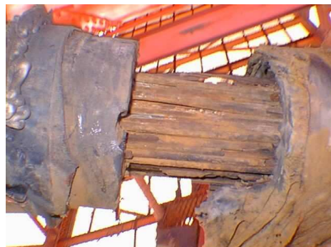
Fig 2 : example of gangrene effect on a PWS cable, Zarate bridge, Argentina
