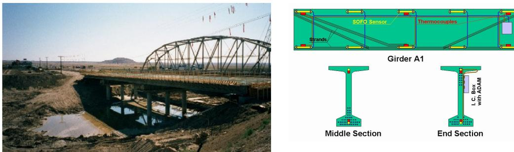
Figure 4. Rio Puerco Bridge view and sensor layout
