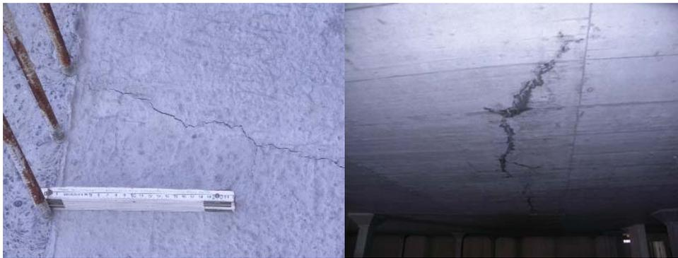
Figure 1. Concrete deck seen from above (left) and from below (right), showing through-going plastic shrinkage cracks.
