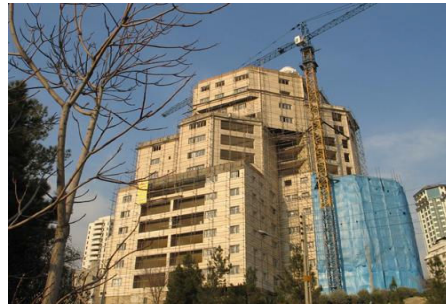
Figure 10: View of building
