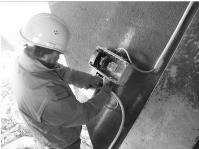
Figure 6. Laser sensor installation
