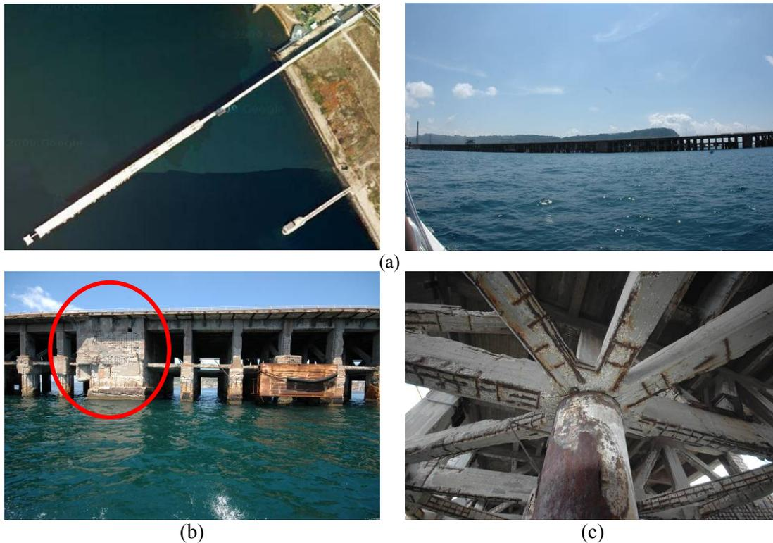
Figure 1. “Pontile Nord” RC pier: (a) global view; (b) caisson; (c) elements of the deteriorated deck structure.
