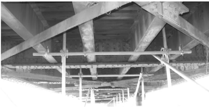
Figure 4. Photograph showing stringers connected to the floor beams
