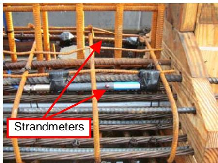
Figure 4. Strandmeters at girder ends (on hairpin bars).
