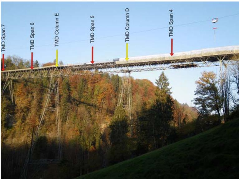
Figure 11, Positions of vertical (red) and horizontal (yellow) TMD's.
