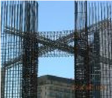
Figure 2. Concrete link beam with diagonal rebar
