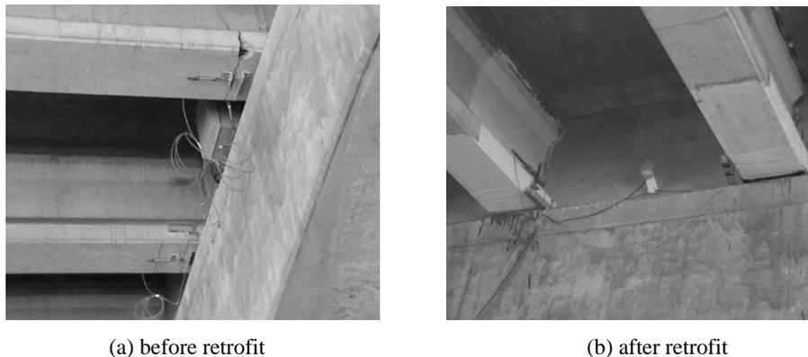
Figure 2. Instrumentation on Beam 6 and Beam 7 before and after strengthening with CFRP.
